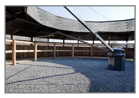
A COLUMBUS open centred roof protects the track and the horses from each weather but allows light and fresh air in so that your horses are not cut of from the outside world. Our open centred roofs are built considering structural engineering calculations according to wind, snow and other environmental influences. All structural details are galvanized and quickly assembled.
