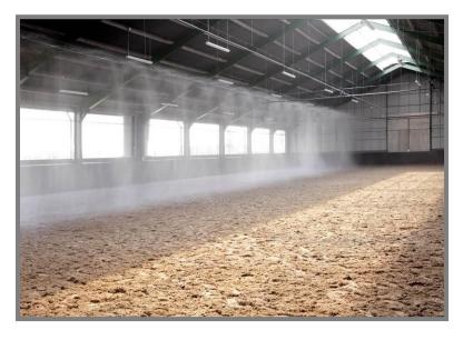
This established system consists of nozzle strands which proceed lengthwise to the indoor arena and are integrated into PVC pipes which are installed on the ceiling of the indoor arena. The nozzles which are installed in approx. 90cm apart from each other nebulize the water evenly. Dust which is in the air will be cohered and the arena footing will be dampened. Our nozzle systems are fitted considering the local conditions and visually integrated into the overall picture of the indoor arena.
